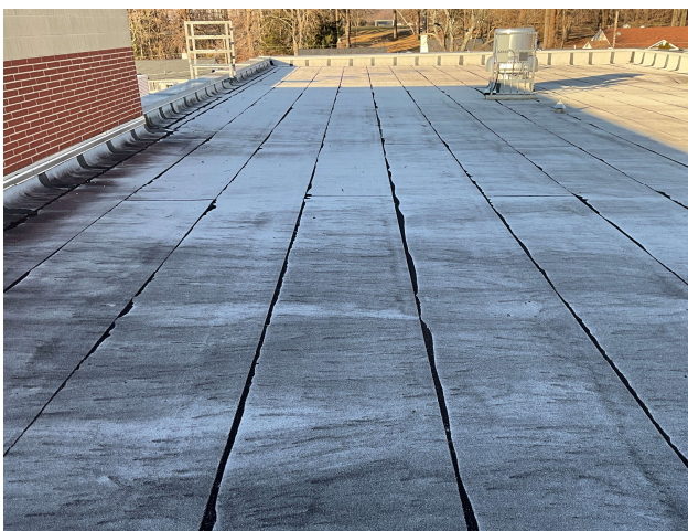
5 - PRIMARY ROOF OVERVIEW
