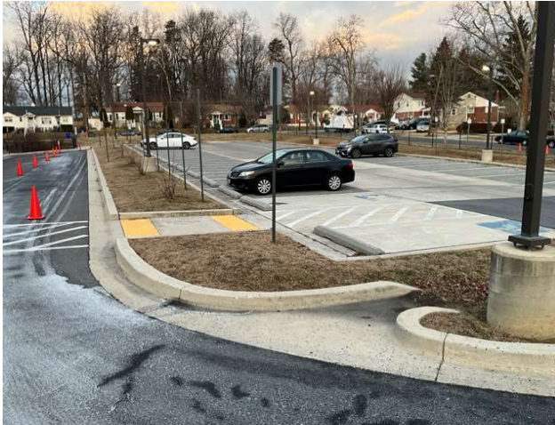
25 - SECONDARY PARKING AREA
