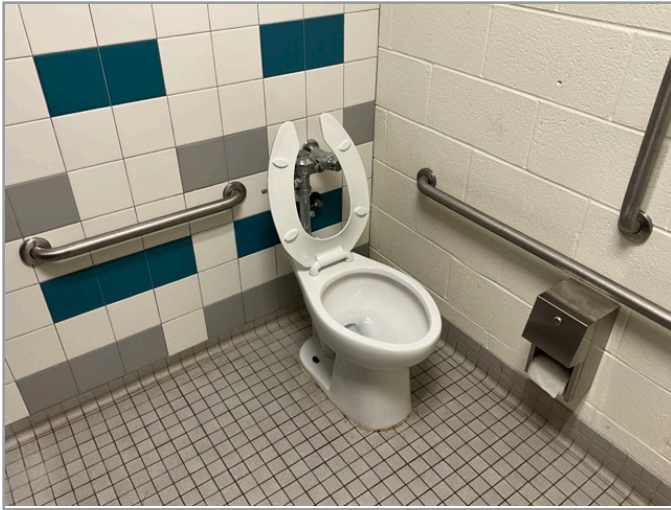
TOILET STALL OVERVIEW
