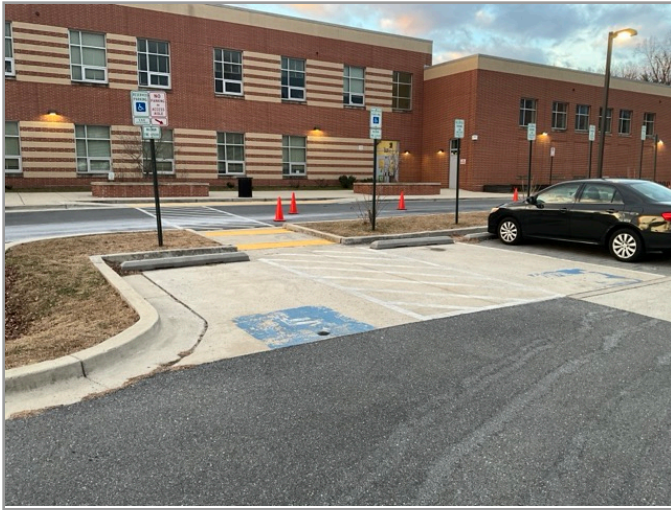
OVERVIEW OF ACCESSIBLE PARKING AREA
